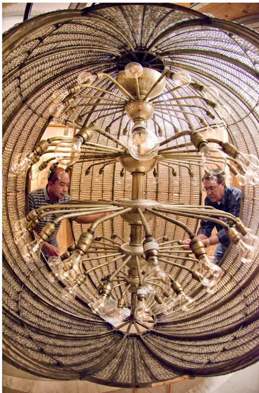
Lighting restorers are shown rewiring the rotunda chandelier in 2012. The large light fixture is six foot in diameter, has 92 light bulbs over 48,000 glass beads and weighs approximately a ton. The chandelier is on an electric winch system that allows for it to be lowered for cleaning and maintenance.
