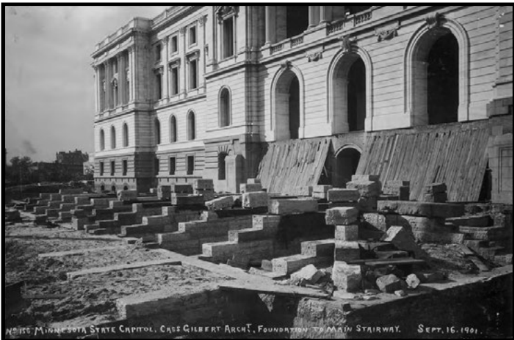
On Sept. 16, 1901 work continued on the foundation of the main stairway to the Minnesota State Capitol.
